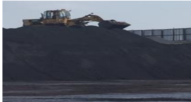
Nahda Coal/Pet Coke Storage Facility
